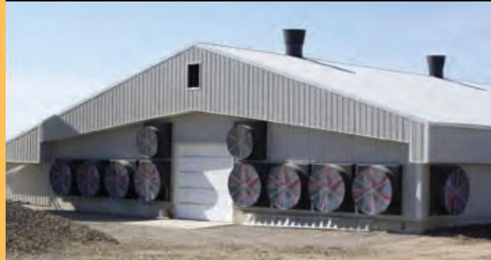
In a typical power ventilation setup, use the Supra to control all fans, heaters, and actuator-controlled ceiling inlets. If you have lights or feed augers that need to be on at certain times, use the Supra to easily operate these. In a farrowing setup, use the Supra's variable stages to control the heat lamps.
