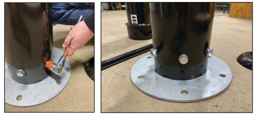
3. Attach upper frame to lower frame using 6 bolts and washers.
