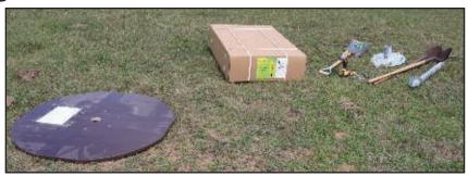
2. Lay base plate on ground and work around edges with shovel
