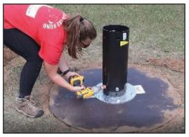
12. Attach upper frame to lower frame using six 16x30 mm bolts and washers
