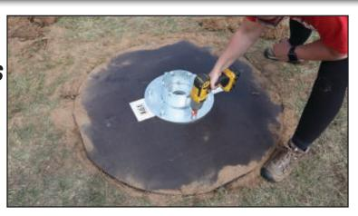
11. Attach lower frame to floor stand using six 16x30 mm bolts and washers and secure
