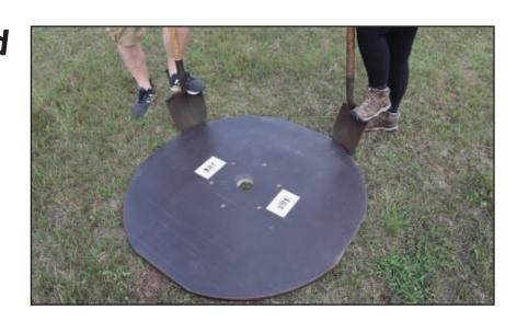
3. Move base plate and dig out area approx. 2-3" deep so base plate will sit just below ground level
