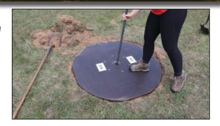
5. Run rod through top hole and begin turning in screw post
