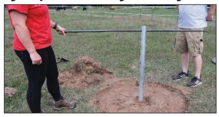
6. Once screw post is securely in ground (approx. 12 to 18") use 16x100 mm bolt to attach TOTEM base attachment to screw post
